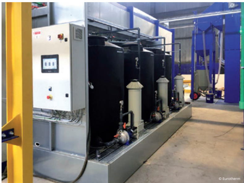
The three water recovery tanks with no discharge to the sewerage system.
